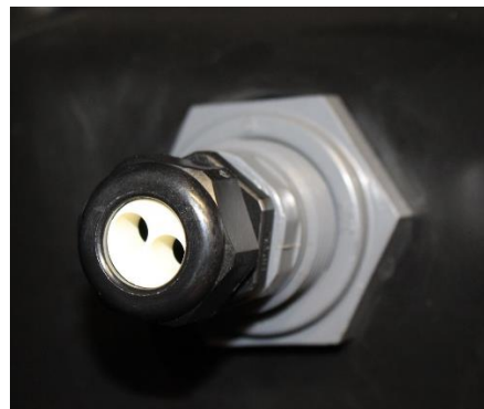
Double gland for level sensor & high level float
