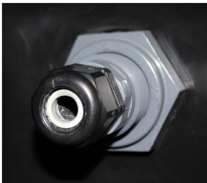
E/One Pump Cable gland
